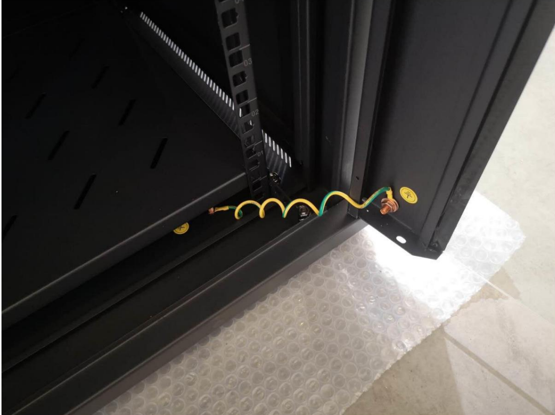
Installation of door grounding as shown in the image.
