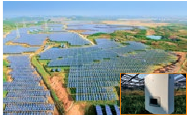
Zhejiang Hangbu Agricultural-photovoltaic hybrid PV plant 30MW
