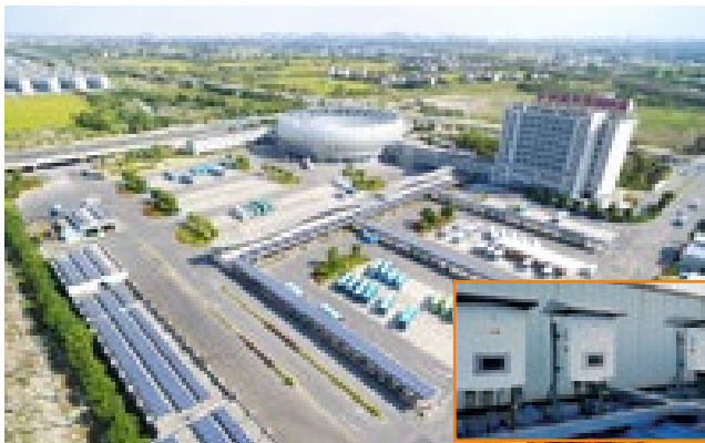
Zhejiang PINGHU Bus Station 472kW
