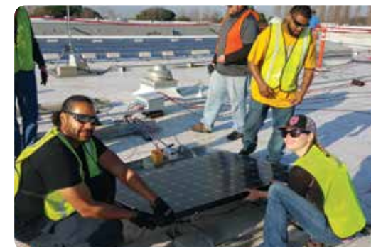
Teamwork to take this roof solar
