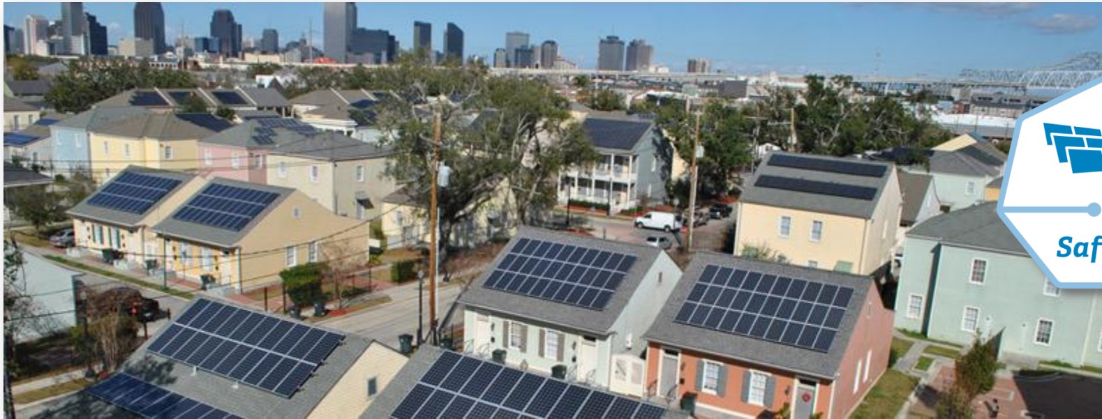
450kW installation on the rooftops of a sustainable neighborhood, New Orleans, Louisiana, USA. Installed by Pontchartrain Mechanical Co.
